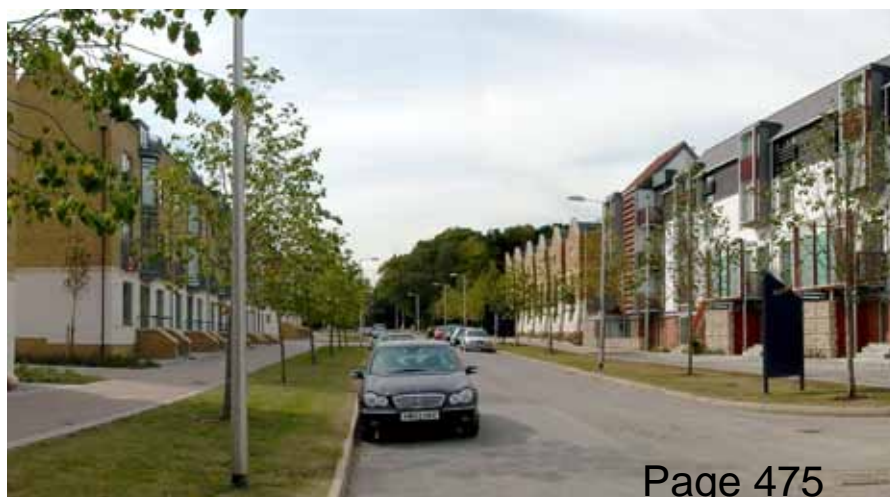
19. Higher densities or taller buildings can be used to positively define key spaces, frontages and main streets. Newhall, Harlow.
